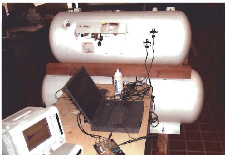
ASCENT's work at VIA includes permanently installing two sonic sensors on the outside of bus tanks in order to verify OPD reliability during fueling. One is located above the 80% fill line, while the second is below.
